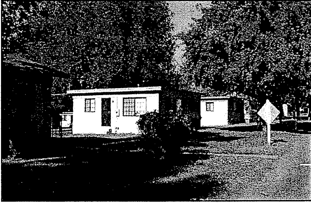
Figure 8. Residences in the Canyon Crest Married Student Housing Complex, formerly a WWII-vintage military housing tract. The two flat-roofed specimens in the center retain more of their historical appearance, but all units in the complex have been significantly altered in recent years.
