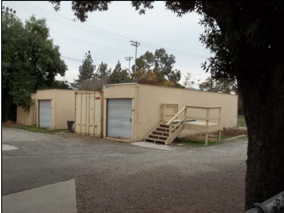
Photograph 3. View of modular units used for maintenance storage.
