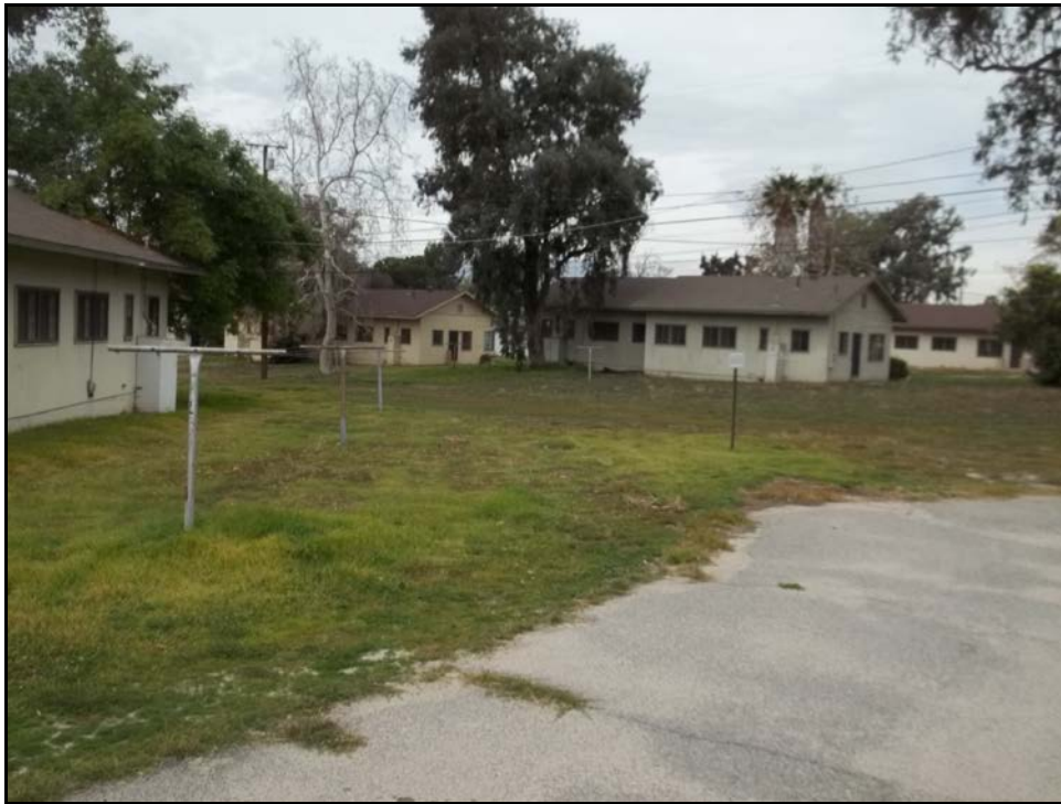
Photograph 1. View of subject site residence.
