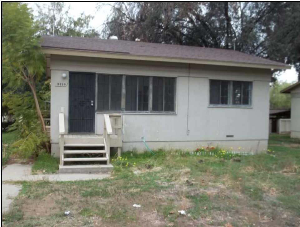
Photograph 2. View of subject site residence.
