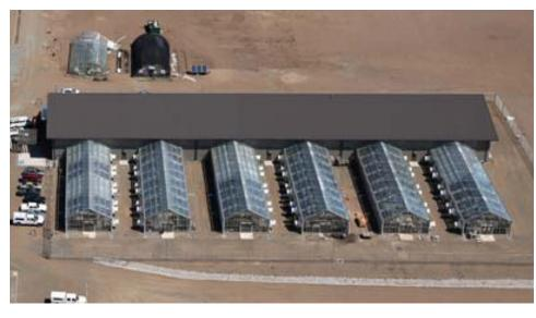
The University of Nevada, Reno was studied at the request of project stakeholders, to gauge the necessity of air conditioning in a desert climate similar to Riverside's. This facility is entirely evaporatively cooled.
