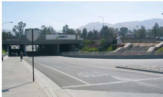
View of Underpass from Lot 30
