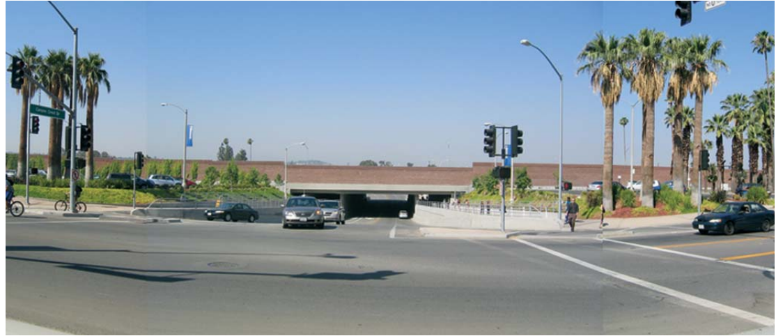
I-215 Freeway From East
