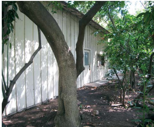
West Side of Barn Stable
