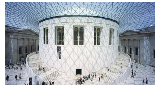
British Museum Roof Addition
