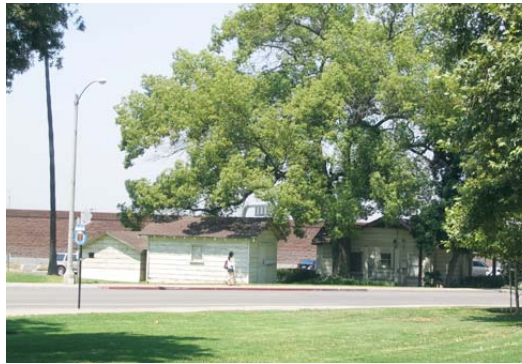
Shed Structure in Lot 4
