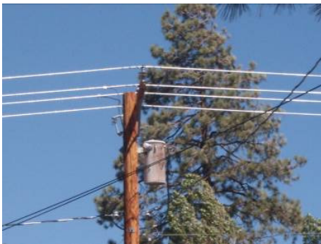
Figure 1: Overhead Transformer
