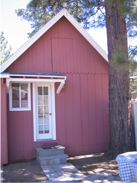
Figure 3: House's South Portion
