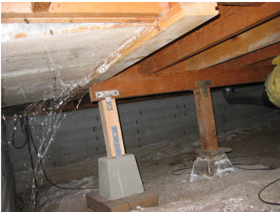
Figure 1: Typical Sub-Floor Construction
