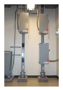
Lighting panel(s) will be provided on each floor that are fed from the busway plug-in circuit breaker(s) which will be equipped with ground fault protection.
