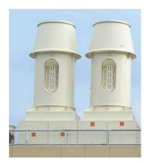
All exhausts will discharge a safe distance above the roof to prevent recirculation through proper dispersion of the air stream into the atmosphere. Discharge stacks will be designed to release the exhaust air at a minimum level higher than any human working on the roof and at a sufficiently high velocity to enable the exhaust air to disperse. The final height, location and discharge velocities will be in accordance with the Wind Consultant's recommendations.
