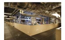
Ductwork from the fume hoods to the linear exhaust valves will be stainless steel.
