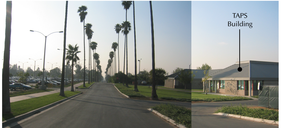
view west down Linden Street
