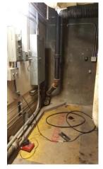
4" and 2" waste and vent stacks at each end of mechanical shaft
