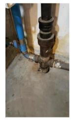
Laboratory waste piped to sanitary waste and vent system using acid waste piping
