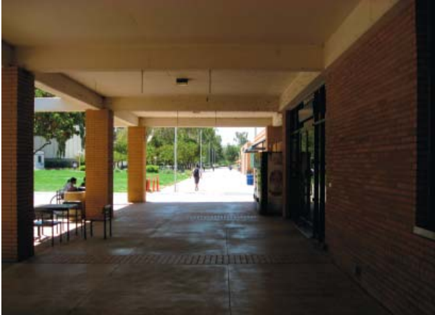
SOUTH COVERED WALKWAY LEADING TO COMMONS MALL
