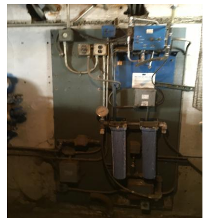
Abandoned distilled water tank
