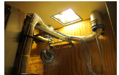
Example for Existing Horizontal Distribution System
