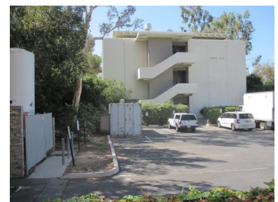
Loading Dock and Service Area
