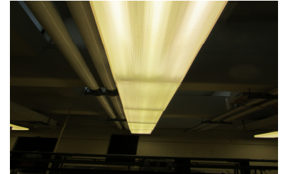
Laboratory lights with discolored lenses
