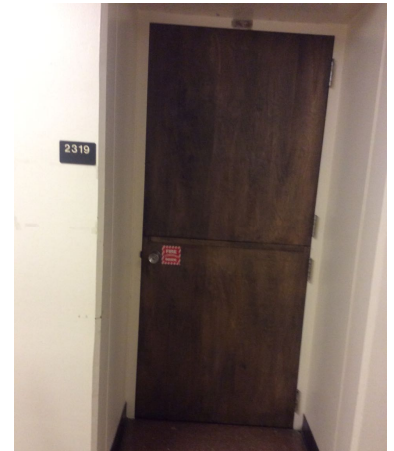
Typical Interior Door
