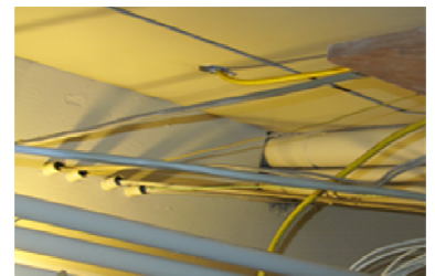
Example for Existing Horizontal Distribution System
