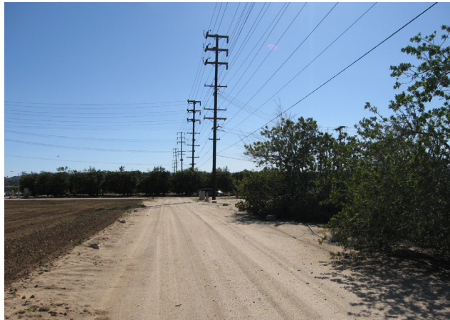
VIEW LOOKING SOUTH FROM EAST SITE EDGE
