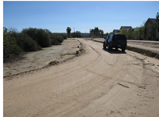
VIEW LOOKING SOUTH ALONG GAGE
